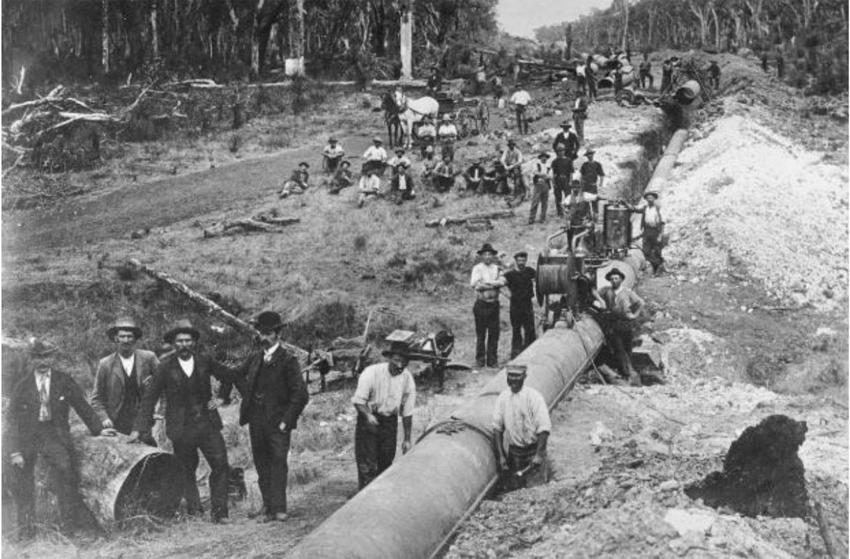
Engineered by C.Y. O'Connor and built between 1898 and 1903, the pipeline delivers water 560 km from Mundaring to Kalgoorlie. It has been a lifeline to the arid interior of Western Australia for more than 100 years and was central to the development of the State.
