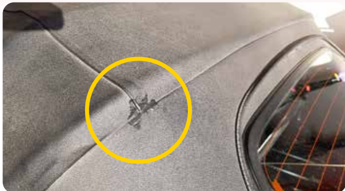
Roof repairs 1 (above) and 2
